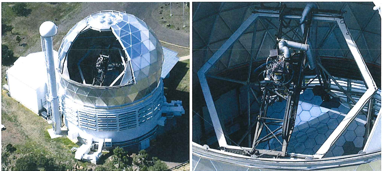
Figure 1. The figure on the left shows the HET pre WFU with the dome shutter open. The figure on the right is a close up view of the top of the HET revealing the primary mirror, and telescope structure which supports the tracker and PFIP.
